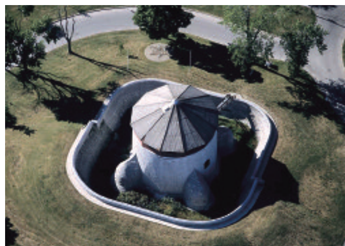
The glacis surrounding Murney Tower is clearly visible in this aerial photograph, 2001, Brian Morin.
