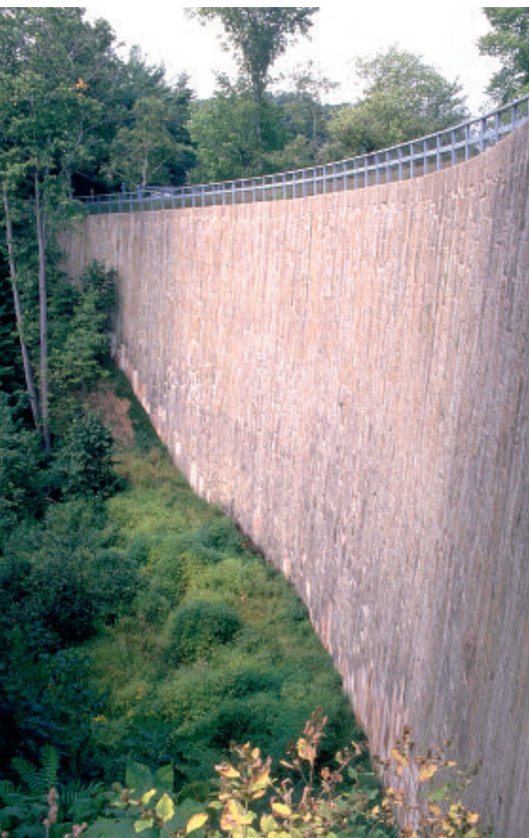
The stone arch dam at Jones Falls was the tallest dam built in North America at the time, 2005, Simon Lunn.
