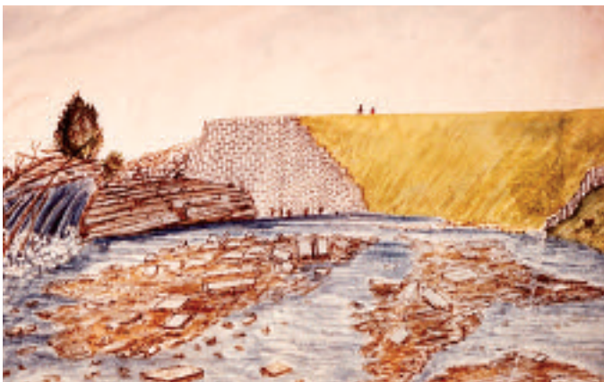
Dam at the Hog's Back showing the Breach in the Stonework 1830, watercolour, Thomas Burrowes, Archives of Ontario.
